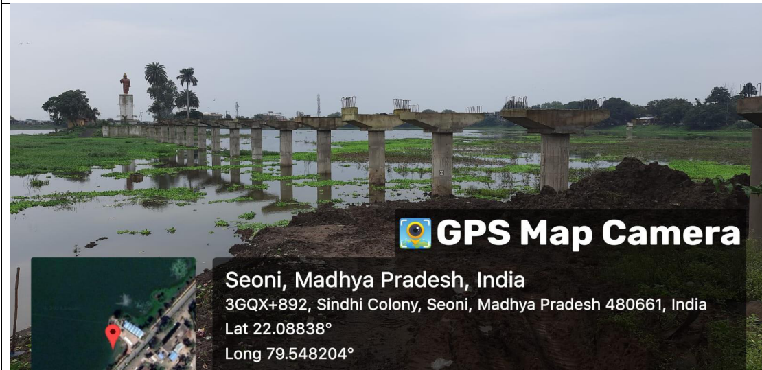
Construction site of Dal SAGR Lake
