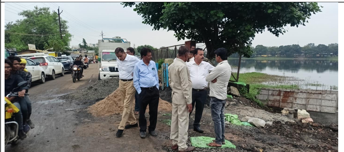
Damaged Lake bund, fencing and pathway
